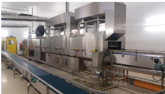
750 TRAYS/HR HOT WASH/HOT RINSE DRY TO 2 GRAMS
